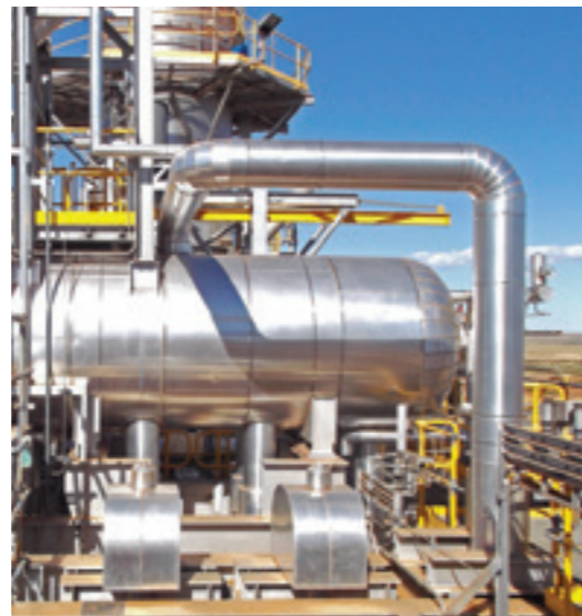
Sino Iron power station, Cape Preston, WA
