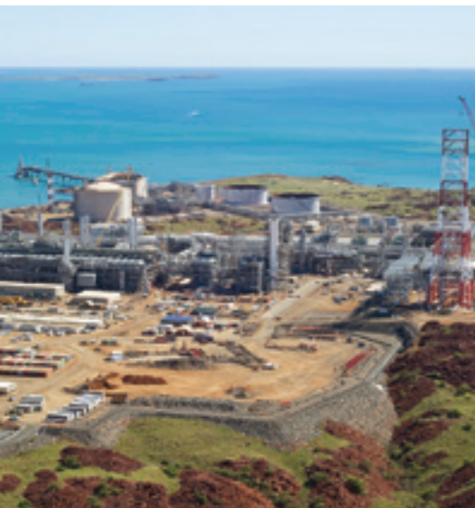
Pluto LNG Project onshore gas plant construction site, Karratha, WA (photo courtesy of Woodside)
