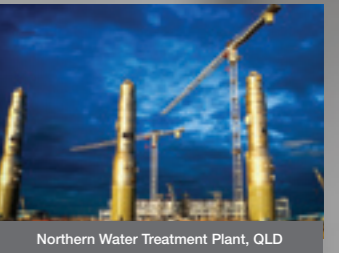
Northern Water Treatment Plant, QLD
