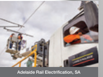
Adelaide Rail Electrification, SA
