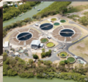
Sandgate WWTP, QLD
