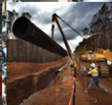
Sugarloaf Pipeline, VIC
