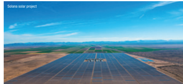
Solana solar project
